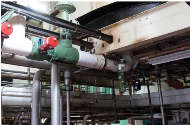
Figure 3. Matt chose the Swirl meter because its piping geometry left little room for straight-run piping to condition the steam flow.
